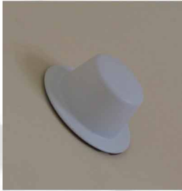
Concealed Sidewall Sprinkler
